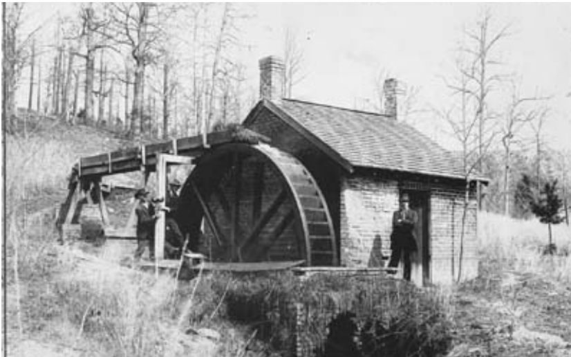
The pump house of the Salem Water Works. (Forsyth County Public Library Photo Collection)
