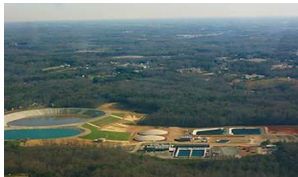
Northwest Water Treatment Plant
