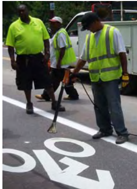
Installing bike lane
