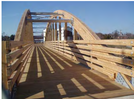
Salem Creek Greenway at the S.E. Gateway Y
