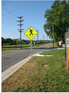
Sidewalks to crossings
