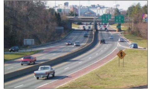
US 52 north of the Stadium Drive Interchange
