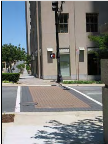
Figure 6: Timed Crosswalk Signal
