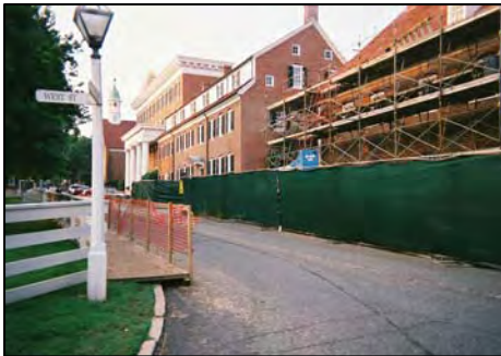
Figure 28: Temporary Sidewalk, Old Salem
