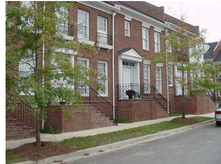
Urban Housing, Vermillion Huntersville, North Carolina
