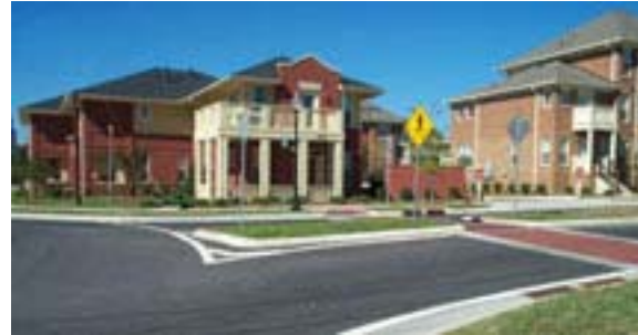
First Ward, Hope VI Redevelopment Charlotte, North Carolina
