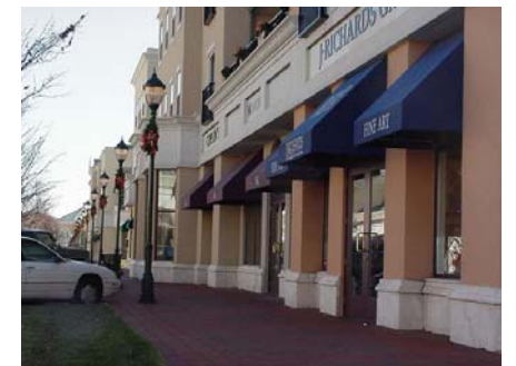
Mixed-Use Development, Phillips Place Charlotte, North Carolina
