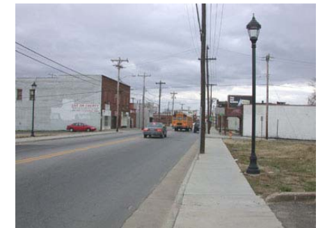
Liberty Street Corridor Infrastructure Improvements
