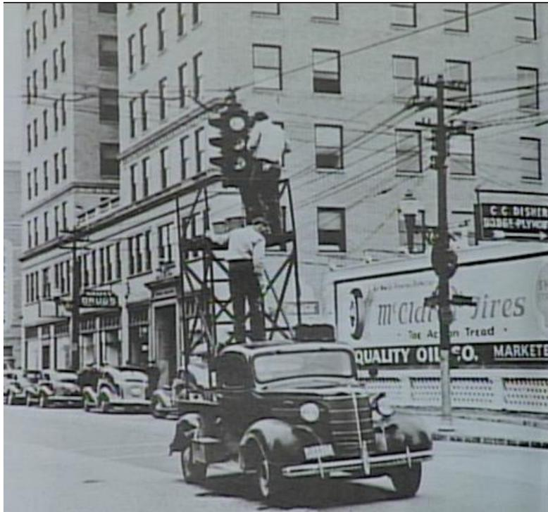
**Before “Cherry-Pickers”, a pickup bed mounted scaffold was used to change burned out traffic lights at 4<sup>th</sup> and Marshall in 1938.** (Forsyth County Public Library Photo Collection)
