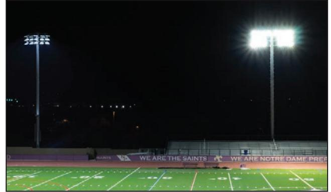
The ordinance requires glare control for LED fixtures for recreation uses and stadiums. The lights on the left side of the image use glare control; the lights on the right side have no shielding.
