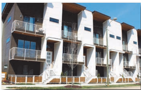
Buildings oriented to a public street with features that help residents feel connected to the neighborhood
