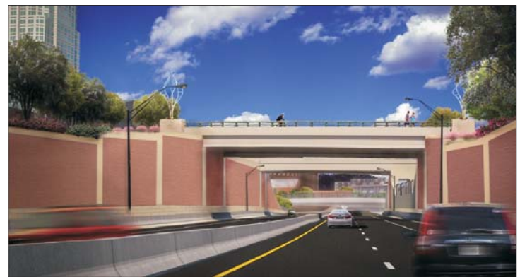
Simulation of brick veneer retaining walls at Marshall Street bridge.
