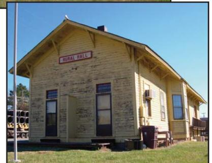
by transoms provide interior access from the north elevation. The building retains some original sliding loading dock doors, but the openings have been infilled with single-leaf doors or twelve-over-twelve sash windows. The six-over-six sash windows elsewhere appear to be original. A bay with three windows projects from the west elevation, and a modern wooden walkway and stairs wrap around the depot's southwest corner.
