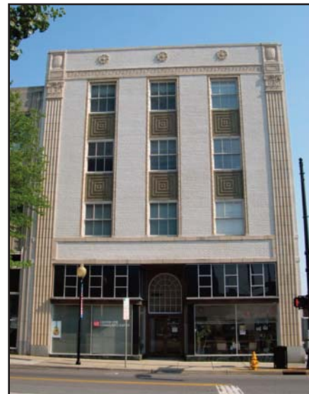
Morris-Early Building, southwest corner of W. Fourth and N. Poplar Streets
