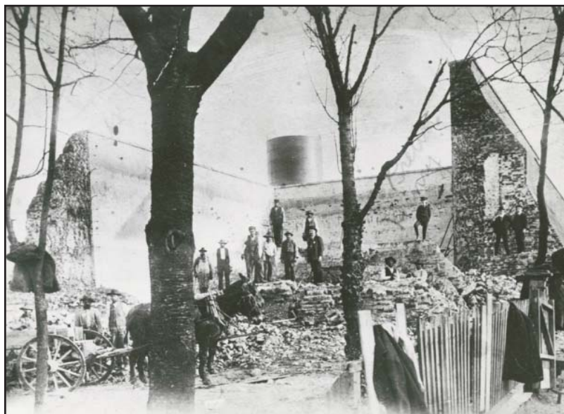
Winston's Water Reservoir after Collapse, 1904 Courtesy of Forsyth County Public Library Photograph Collection
